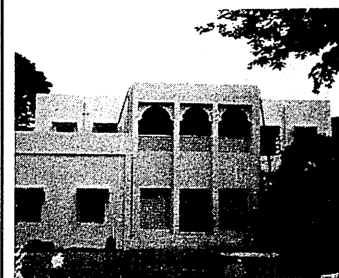
Claybrook no longer looks like what it used to be in the days Binny's executives occupied it. Now the main building of the Bharatiya Vidya Bhavan's Rajaji School, it has seen quite a bit of alteration in recent years and is as shown in the picture.
