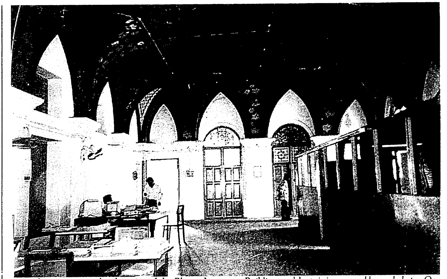
Bradma occupy a palatial portion of the Bharat Insurance Building and keep it in reasonably good shape. One skylight still retains its original stained glass (below) but the other has ordinary glass where stained glass once used to be. This room has a magnificent, semi-vaunted wooden ceiling. (Pictures here and on page 1 by RAJIND N CHRISTY.)
